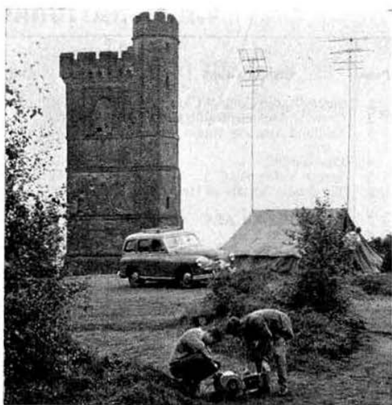
Dorking and District Amateur Radio Society had their 'B' station on Leith Hill, famous Surrey landmark at 997 ft. a.s.l. For 70 cm, a corner-reflector built by G3OVS gave good results, whilst for 70 Mc/s a 4 element Yagi was used. Here, SWLs Ron Hodson and Peter Gilbey stoke-up the generator, whilst G3HJZ steers the 4m beam.
